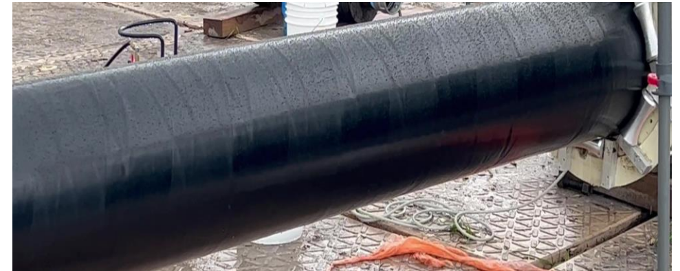
1.3-mile-long, 16" IHC installed at 8 ft./min. during pilot program with strategic partner.
